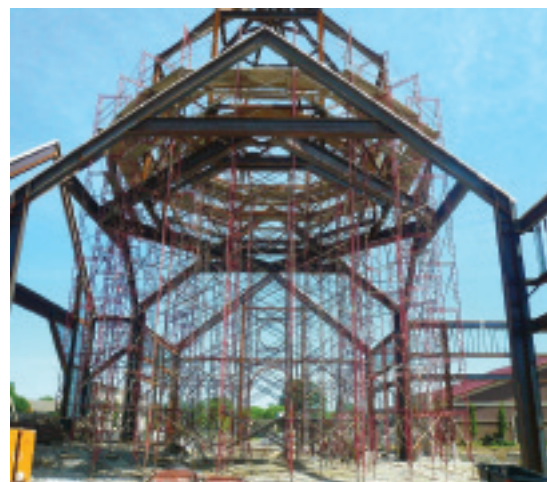
A Waco Scaffolding & Equipment job at a church in Westerville, OH.
