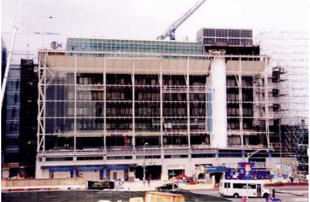
The southern end of the construction, called "the sleeve," is a glass wall supported by tubular truss and adjustable cables.
