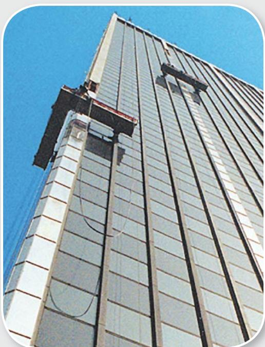
Corner sections can be used to follow the contours of the structure precisely and allow access within 30 to 60 cm. of the working surface. You can choose from a variety of fixed and adjustable corner sections.
