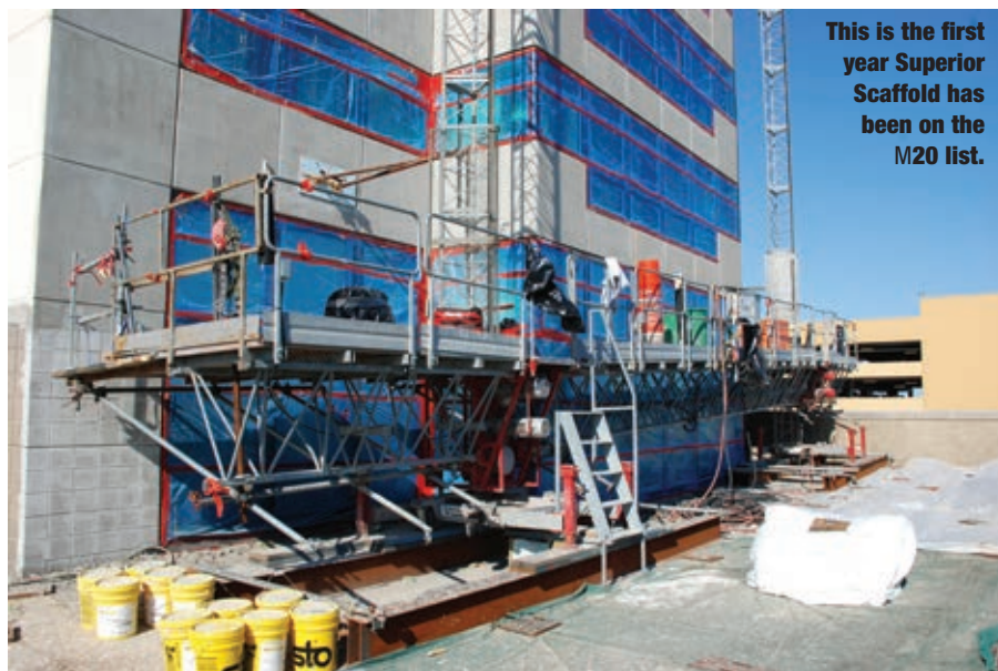
Marr Crane & Rigging provided installation and dismantling services for the Hydro Mobile units, seen here.
