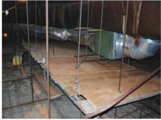
This job was done entirely using suspension. We used beam clamps with tubes to anchor to steel when we could. We also used standard drop-in cement anchors to hold the cables when there was no steel to tie-in to. There was very little room for error — or bodies for that matter.
