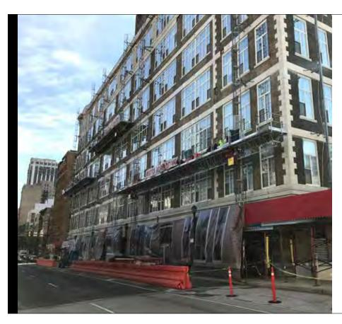
The renovation is a year-long project with the next phase just beginning. The mast climbers will be moved to the west and east sides and then eventually to the south side, where the work will finish.
