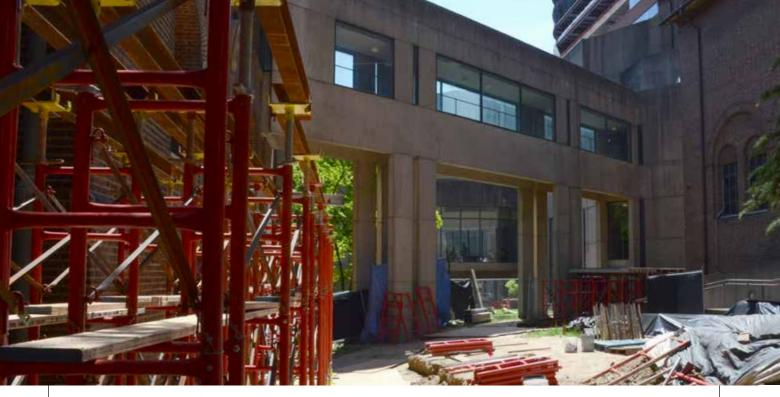
They then built an exit ramp out of system scaffold in order to elevate the Sphinx enough to get it through the window.
