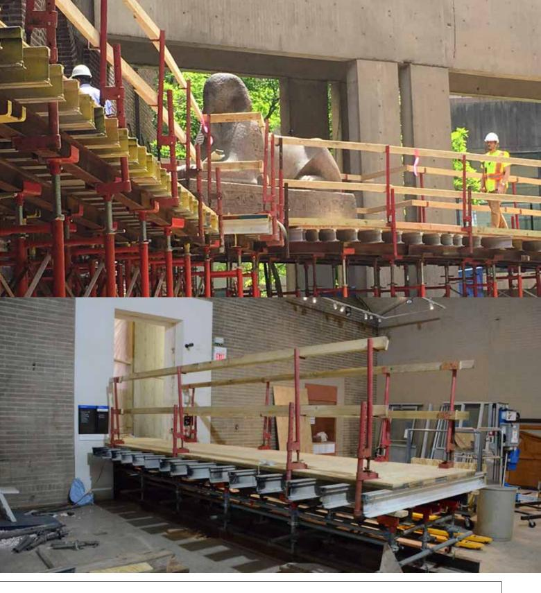
entire route. It took some creative layout to position the shoring frames around several pipes at the back end of the ramp. The final step in preparing access was to build another deck or loading platform out of system scaffold on the inside at the other end of the long ramp to receive the
